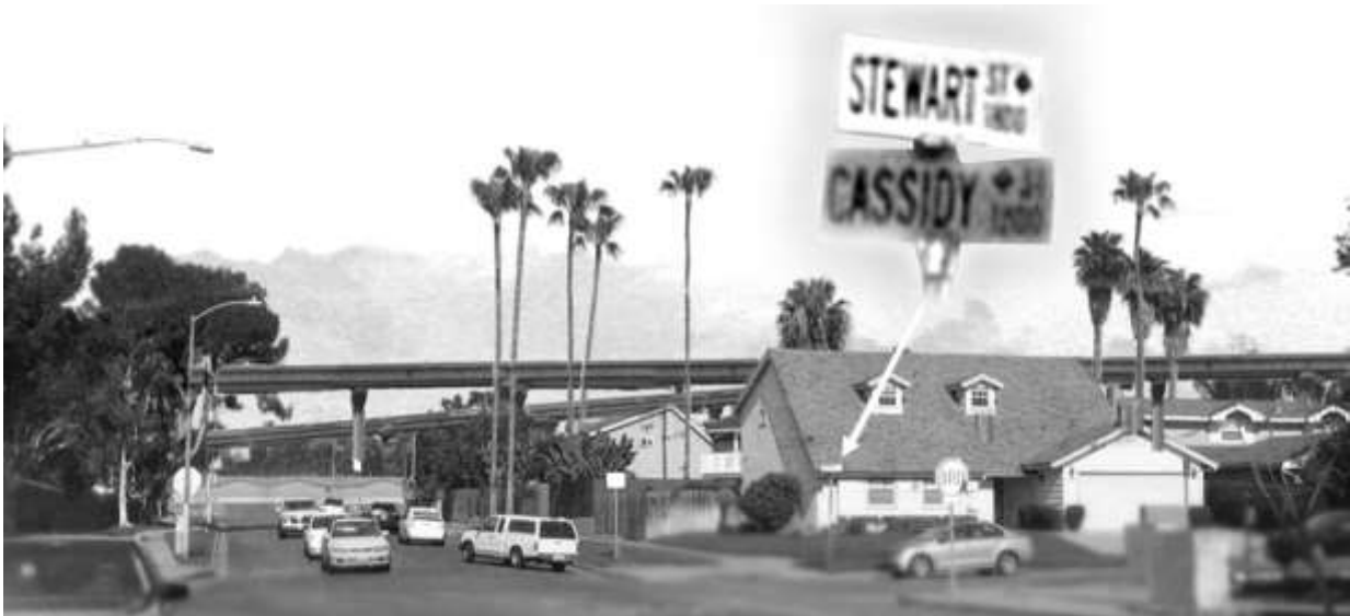
Figure 2 Proposed Western Flyover Lane, Serving an Expanded I-5 – SR-78 Interchange, Looking East on Cassidy, From Across the Street from South Oceanside Elementary School
